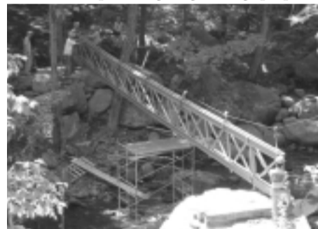
The 1,500-pound section is "flown" into position.
