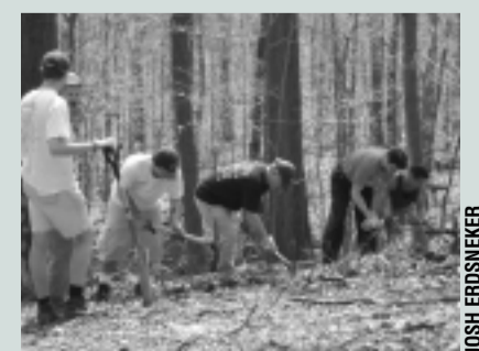
Volunteers get hands-on training at the Trail Construction workshop.
