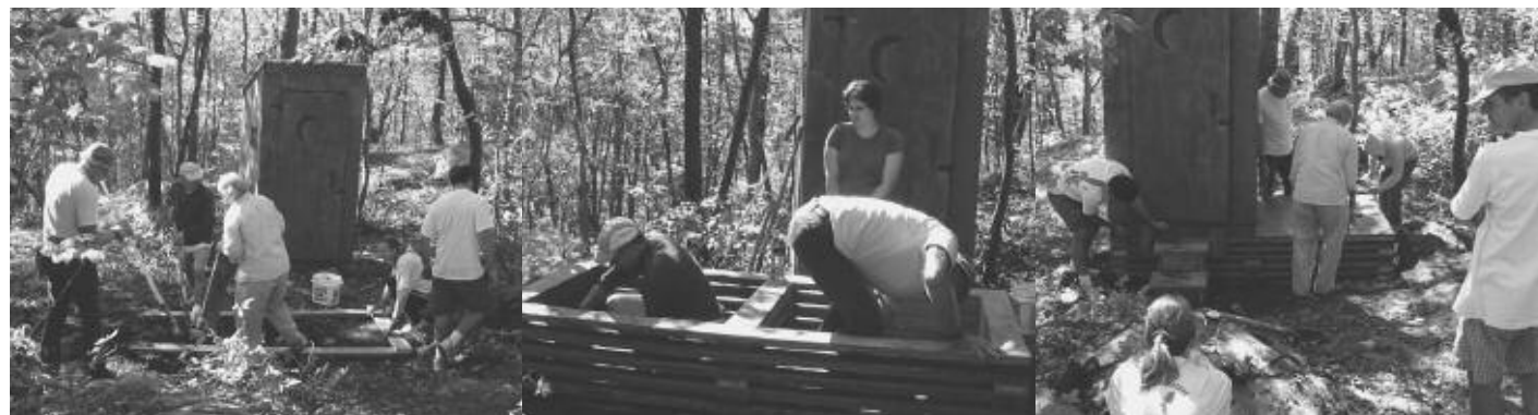
The team levels the base and starts building the crib.
