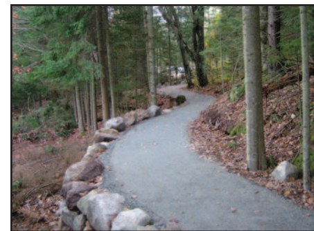
Example of stone cribbed tread for ADA trail, a recommendation for Van Cortlandt Park.
