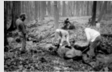
Heavy lifting by the West Hudson Crew.
