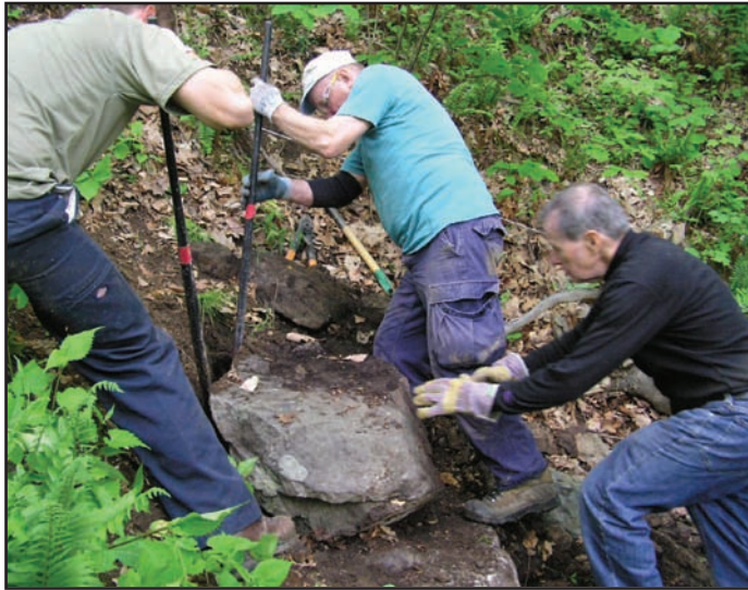
West Jersey crew members work a step into place on the Warren Trail.
