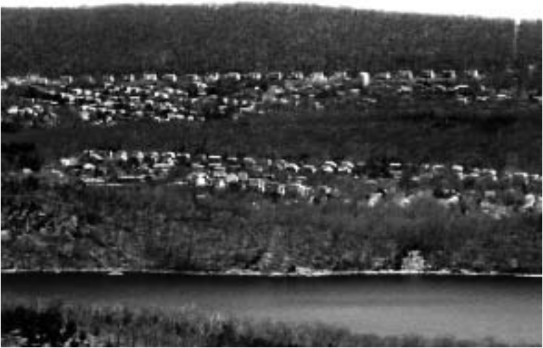
Townhouse development along Skyline Drive, on the west slope of Ramapo Mountain, seen from Wyanoĳie High Point.
