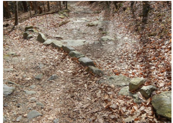
Mr. GOOD BAR: Water easily sheets off the trail thanks to the 45 degree angle of this bar.
