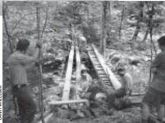
Old and soon-to-be-new bridge, side by side over the Flatbrook.
