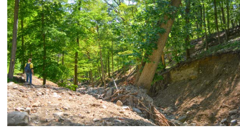
Major trail washout in Bear Mountain State Park
