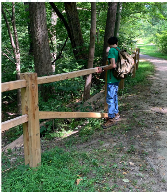
Andrew repairing the fence along the OCA
