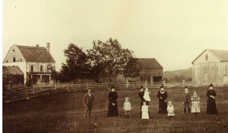
The Ryerson House on Hook Road, with the Drew family in front. The site is now entirely beneath the Wanaque Reservoir. Photo courtesy of the DeBenedetto Collection, Wanaque Public Library
