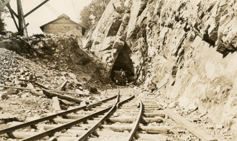
Railroad tracks were laid to carry materials during the construction of the reservoir. Photo courtesy of the DeBenedetto Collection, Wanaque Public Library
